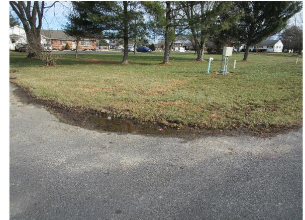
Parking spaces in the parking lot can be converted to porous pavement to capture and infiltrate stormwater runoff from the parking lot and rooftop. A rain garden can be installed in the turfgrass area east of the parking lot to capture, treat, and infiltrate stormwater runoff from the parking lot. A preliminary soil assessment suggests that the soils have suitable drainage characteristics for green infrastructure.
